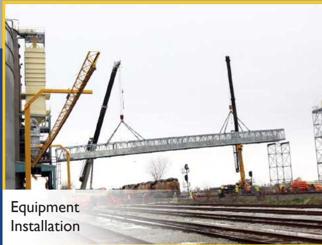
Support Tower Installation
